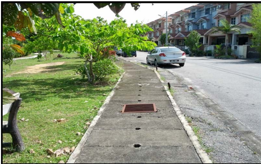
Gambar 2: Contoh parit tertutup saiz 1200mm
